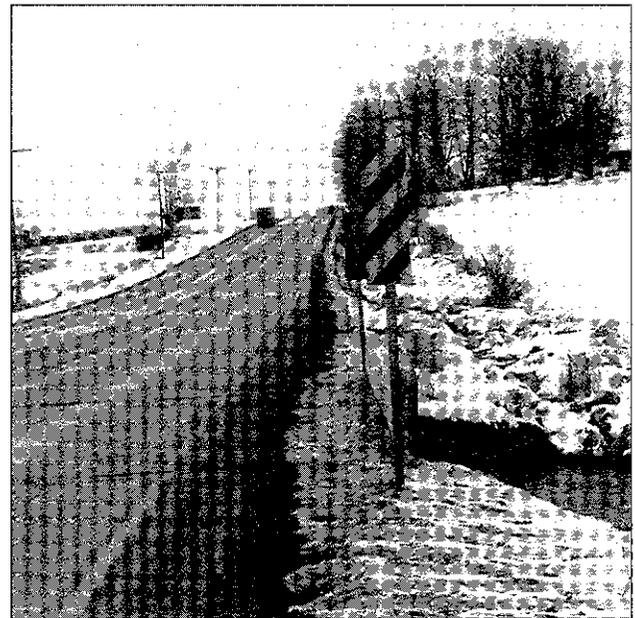
The photo at the left is an example of a bridge rail/culvert head wall that a driver might not see at night or in rainy weather. The driver could hit it, or when becoming aware of it, abruptly turn into the other lane. The photo at the right demonstrates how effective object markers can be in warning a driver of the potential hazard.
